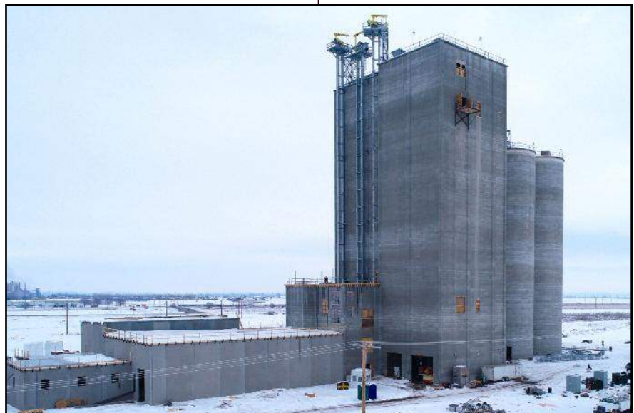
Southwest elevation of Fremont, Nebraska, feed mill facility
