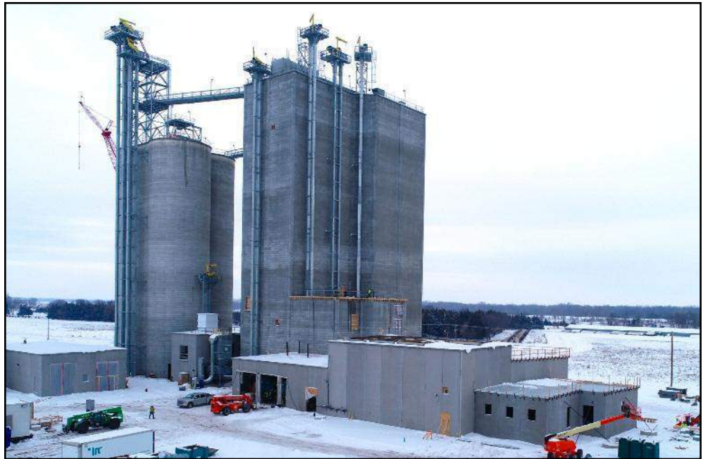
Northwest elevation of feed mill facility
