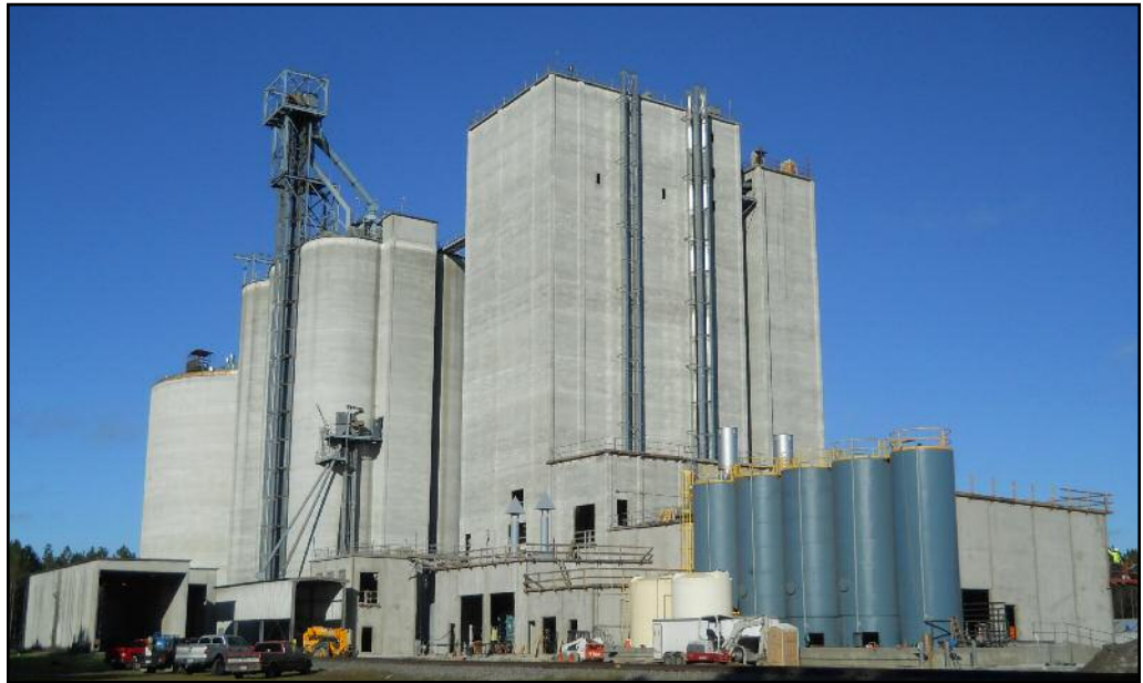
Left to right: Existing receiving building, 100-foot-diameter silo, existing 6-pack grain storage, feed mill, warehouse, and tank farm
