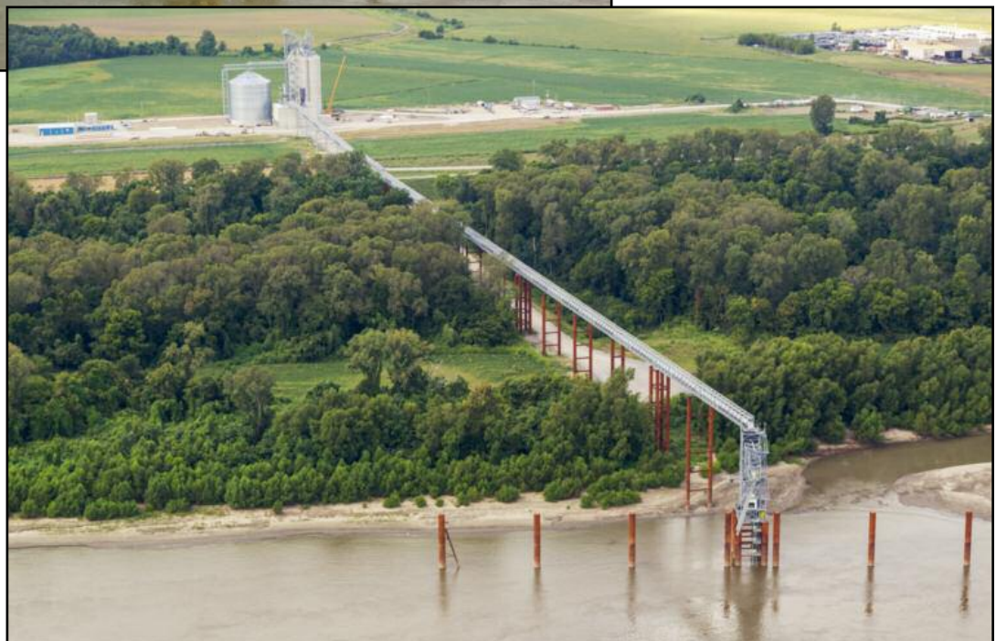
Above: Barge surge hopper tower and barge loadout spout tower
