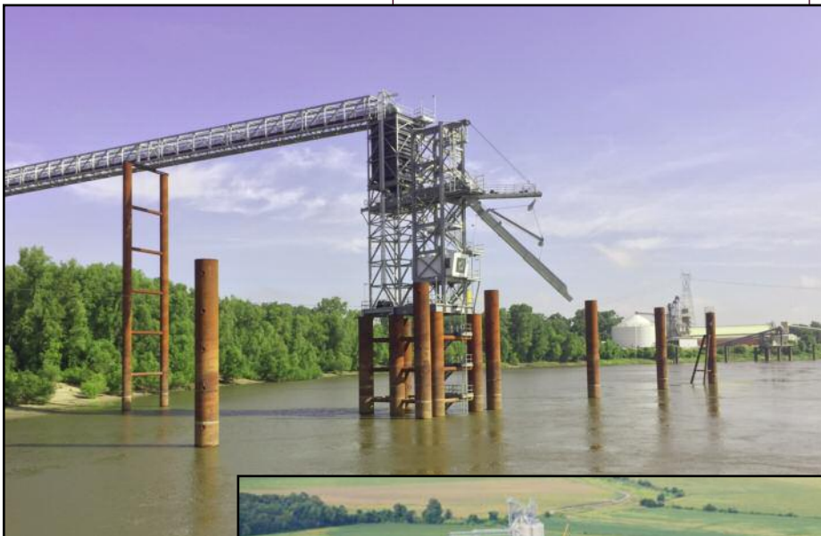
Above: Barge surge hopper tower and barge loadout spout tower
