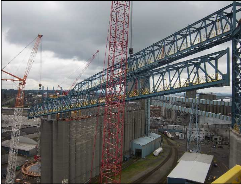
Second 300-foot bridge being lifted into position
