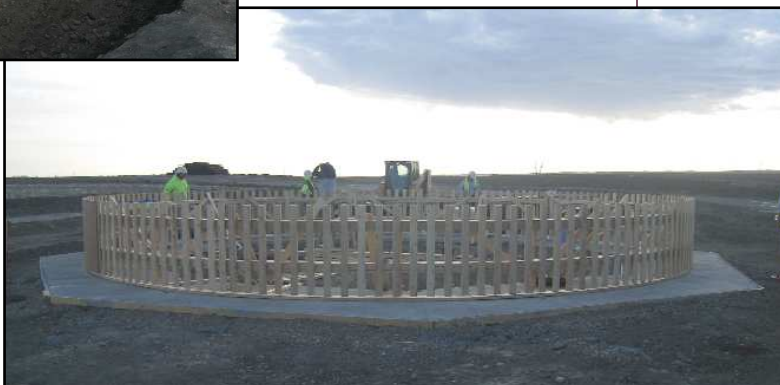
Right: 35-foot-diameter slip form being built at the Conrad site
