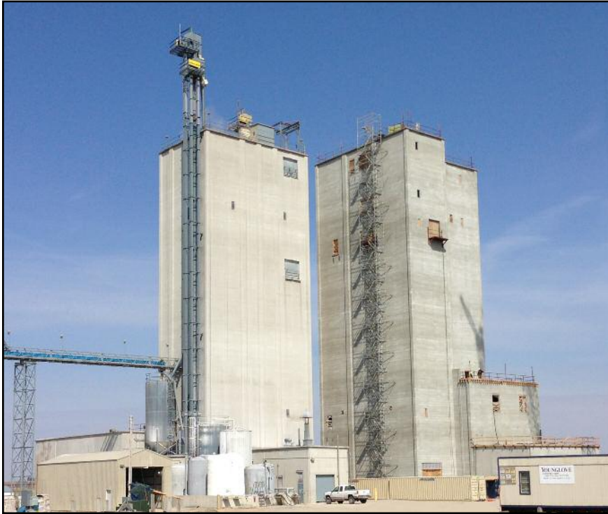
Exterior view of Mill 1 (left) and Mill 2 (right)
