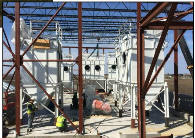
Right: View of structural steel at penthouse
