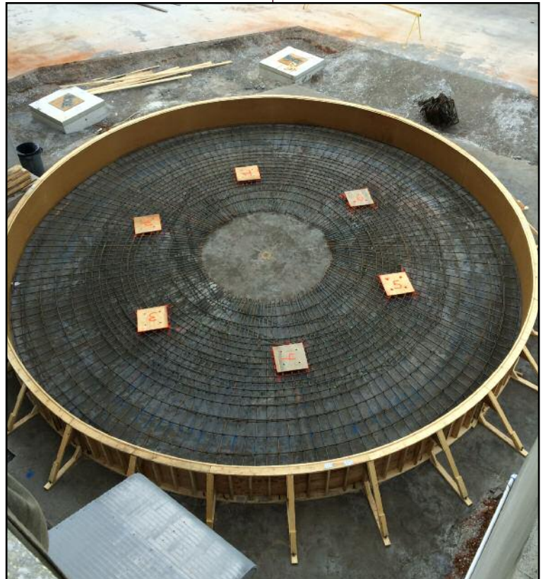
Mat slab rebar placement
