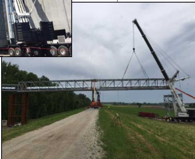
Above: Setting the conveyor bridge over the 92-foot-diameter steel tank
