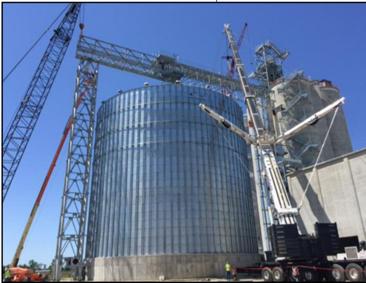
Above: Setting the conveyor bridge over the 92-foot-diameter steel tank
