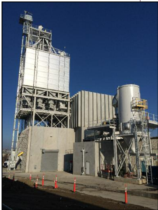
Receiving driveway with bulk storage bins above
