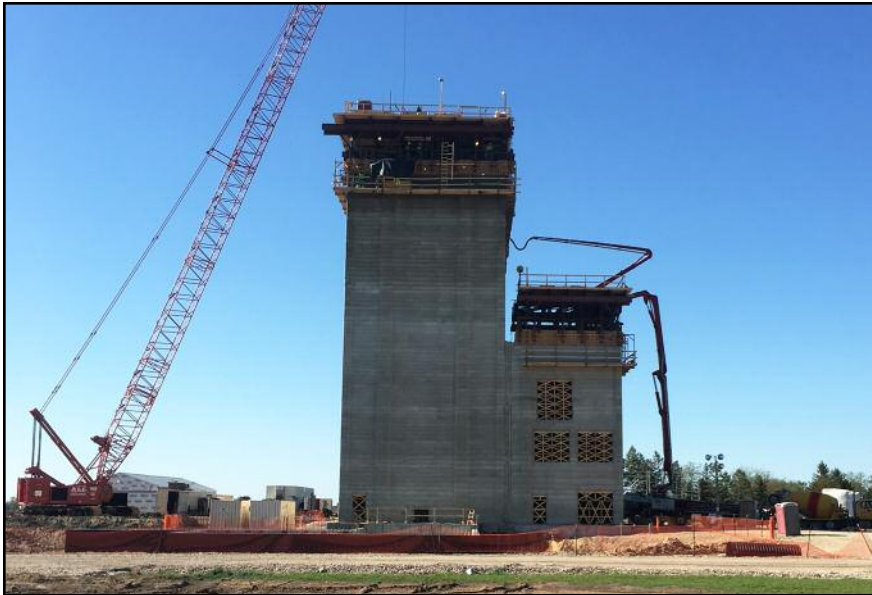
Day 4 of the slip (view looking south)
