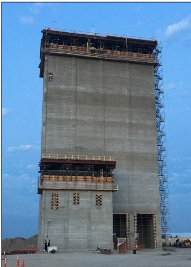
Day 7 of the slip (view looking east)
